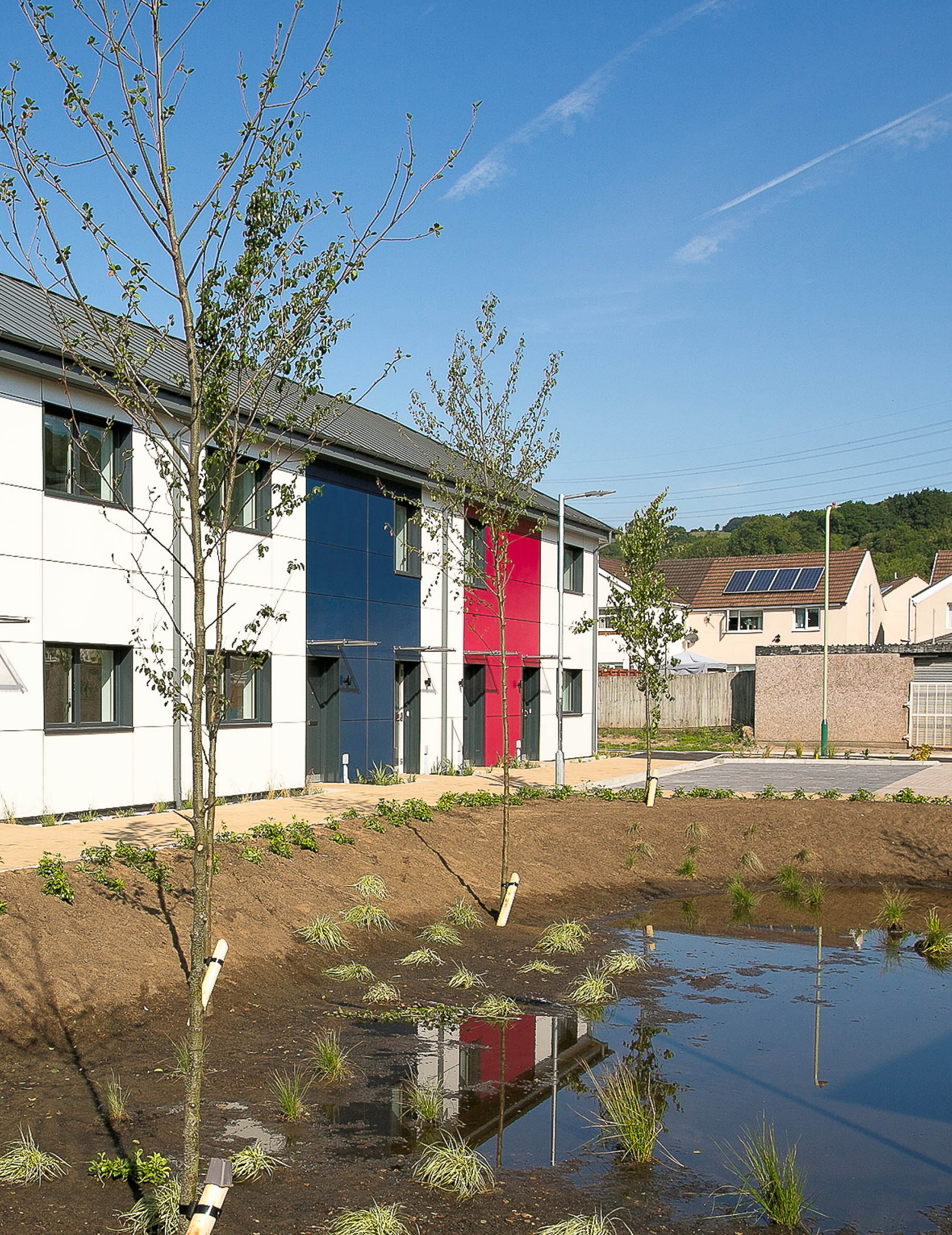
Recently completed houses and apartments in Trethomas and Trecenydd, for Caerphilly County Borough Council. Designed to Passivhaus standards.
