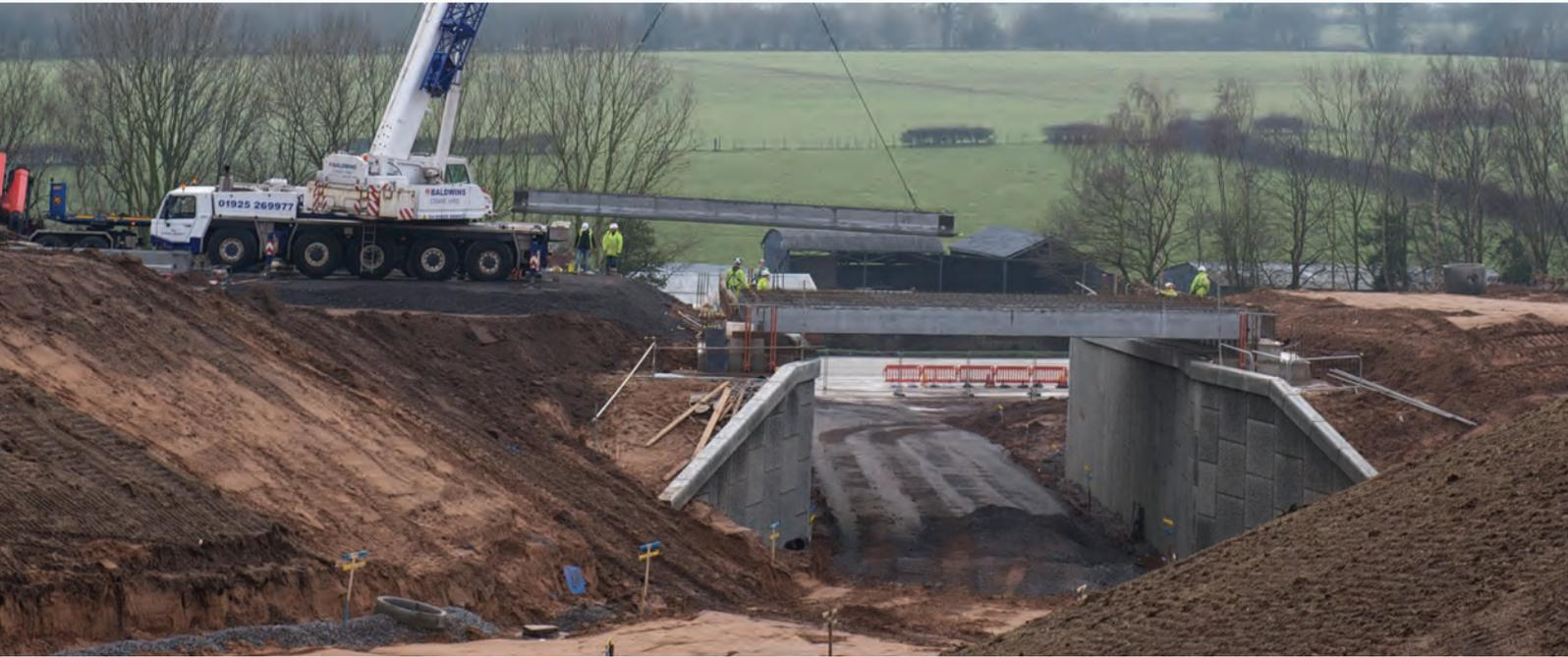
The Wrexham Industrial Estate Access Road is a Welsh Government-funded highway scheme providing improved access to one of the largest industrial estates in Europe. The scheme involves the construction of 4.4km of new highway with two reinforced concrete overbridges and a number of culverts, as well as dealing with a high concentration of existing services that require diverting.
