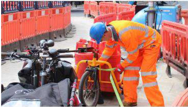
Delivering hydrogen cylinders to the TfL Highbury Project
