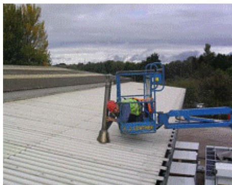
Using MEWP to inspect a vent
