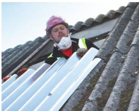
Replacing roof-light from below
