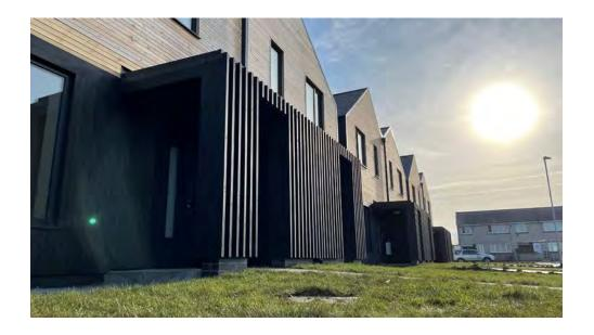
This project for Isle of Anglesey County Council centred on the provision of social housing constructed offsite using an innovative modular approach. It is the first multi-unit housing scheme to be manufactured and built in Wales using such a technique – and the first to be delivered using Welsh timber.
