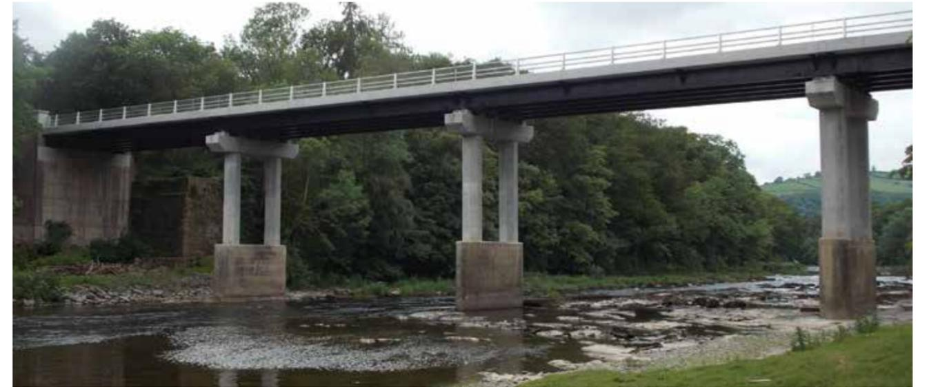
The project involved refurbishing a bridge over the environmentally sensitive River Wye while keeping the bridge open for people cycling or on foot. The client, Powys County Council, and Natural Resources Wales (NRW) had planned the use of hydrodemolition to remove the bridge's existing concrete, but Dawnus, the main contractor, believed this presented a serious environmental risk.
