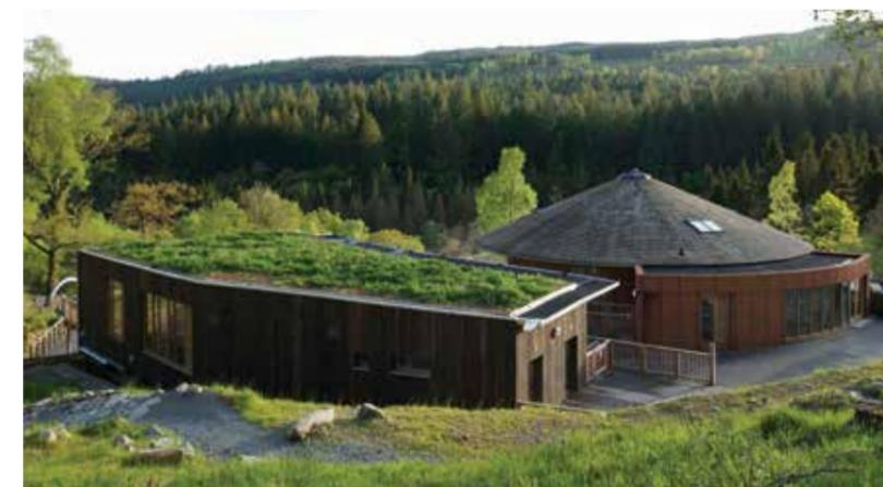
Set in the Snowdonia National Park, this visitor centre is the first in the UK built from low-grade local timber and manufactured Brettstapel. The pioneering project used off-site fabrication to minimise the environmental impact, improving productivity and shortening timescales while respecting the beautiful surrounding landscape.
