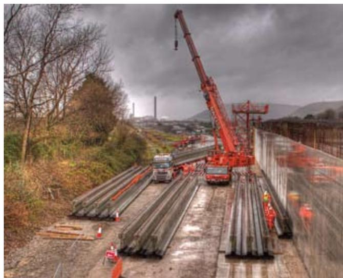
There was an additional environmental impact from this collaboration, as slag from the blast furnace at the steelworks is sold as a by-product. It was used to provide more than half the 400,000m<sup>3</sup> of material needed to build the embankment on which the road was being built. Apart from the recycling benefits, the proximity vastly reduced potential lorry
