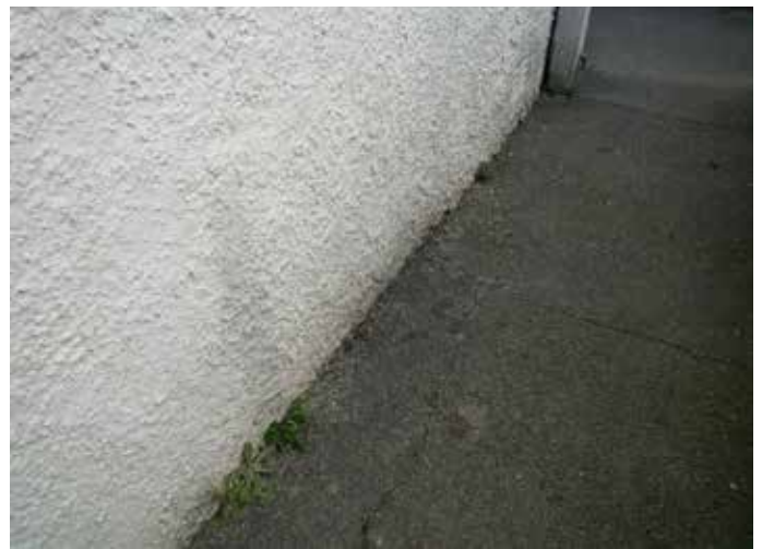
Figures 25 & 26: showing render to ground formation level at the rear of the property, and no weep holes
