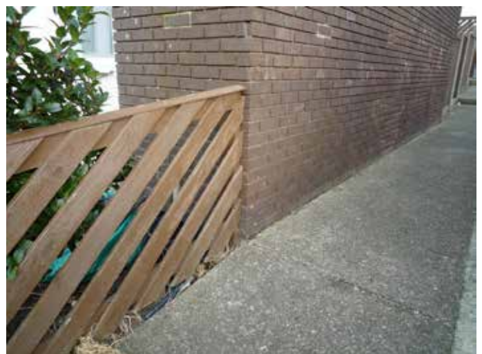
Figure 55: Typical fencing abutting main walls prior to EWI installation
