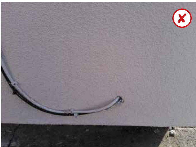
Figure 38 – cable clipped
