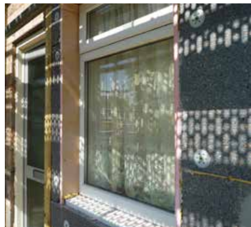
Figure 58: Insulated reveals and head
