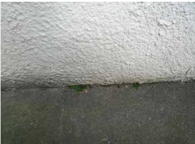
Figures 25 & 26: showing render to ground formation level at the rear of the property, and no weep holes
