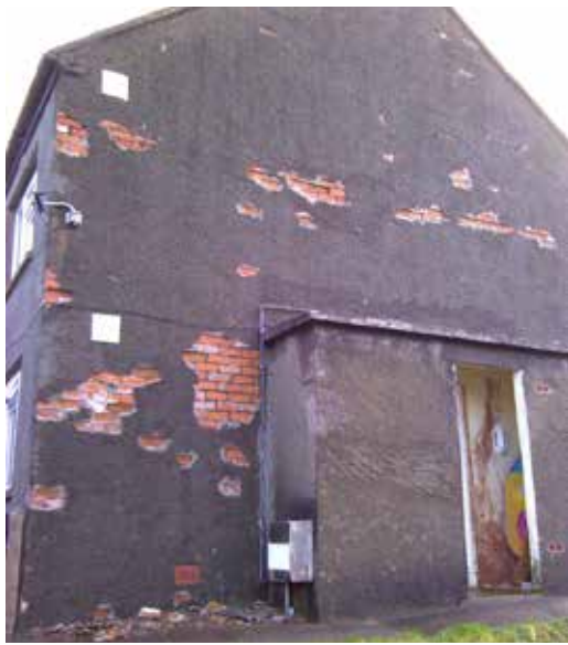
Figures 29 & 30: Gable end wall damage caused by saturation and blown render
