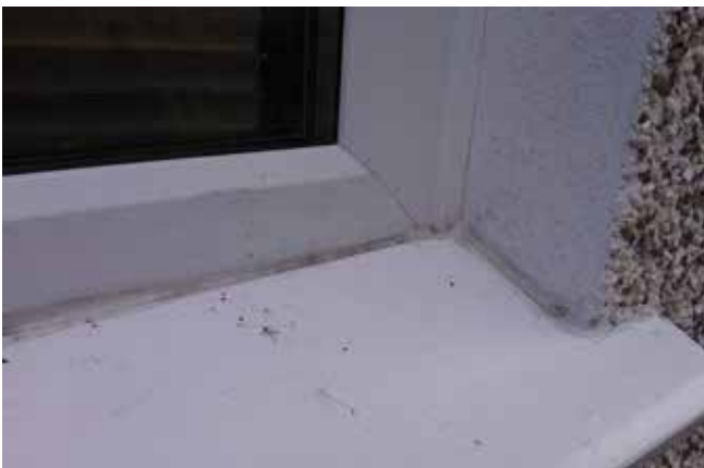
Figure 31: Uninsulated window reveal
