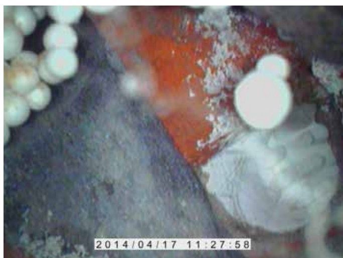
Figures 23 & 24: Missing insulation below rear kitchen window and rear bedroom window
