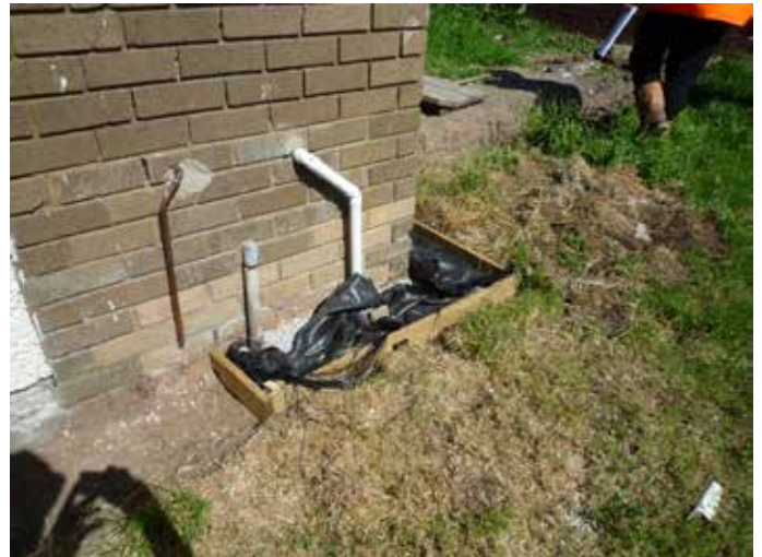
Figure 54: Ongoing works to provide soak away on raised ground areas.
