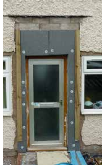
Figure 56: Porch removed and cold bridge removed
