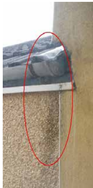
Figure 43: poor detailing
