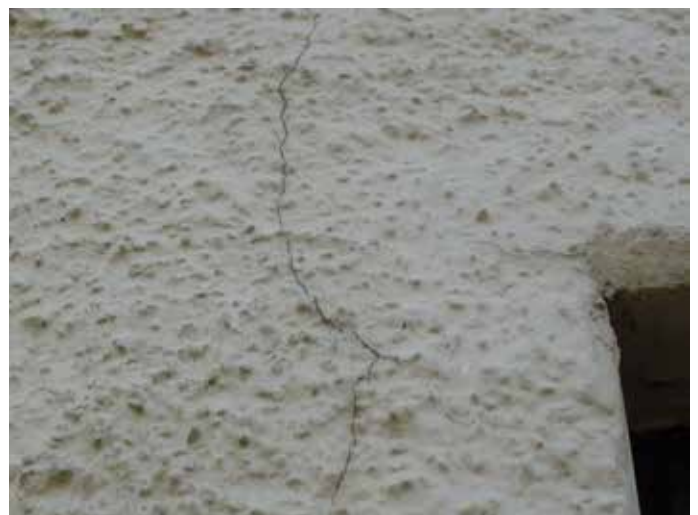
Figure 28: Cracked render at the property
