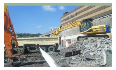
Derwen Group recovered more than 20,000 tonnes of inert materials and supplied over 5,500 tonnes of material recycled to the Quadrant site for use as general fill and subbase with the remaining 15,500 tonnes sold by Derwen Group for other construction projects. In addition, 5,000 tonnes of tarmac and concrete material was reprocessed and reused in situ.
