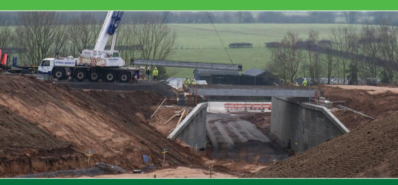
The Wrexham Industrial Estate Access Road is a Welsh Governmentfunded highway scheme providing improved access to one of the largest industrial estates in Europe. The scheme involves the construction of 4.4km of new highway with two reinforced concrete overbridges and a number of culverts, as well as dealing with a high concentration of existing services that require diverting.
